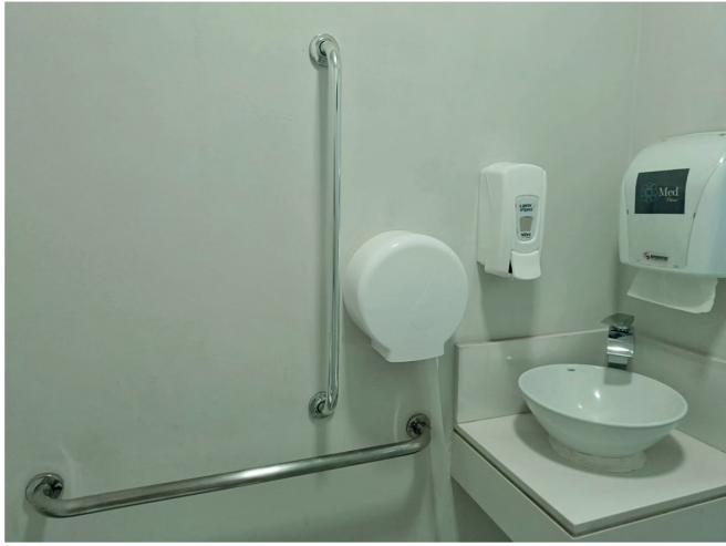
Figure 5. Sink countertop with free lower space for better accessibility.
